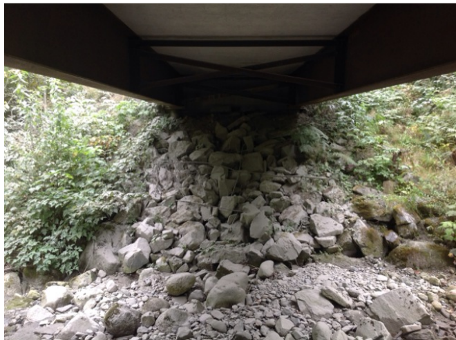
Right Bank Abutment when facing downstream
