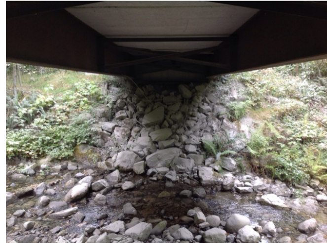
Left Bank Abutment when facing downstream
